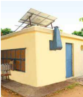
CIPHET evaporative cooled storage
