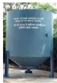
Paddy straw based biogas plant
