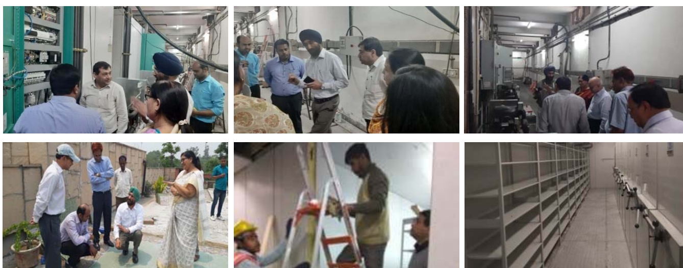
Fig. 6.4. Work in progress for upgradation /modernization of National Genebank
